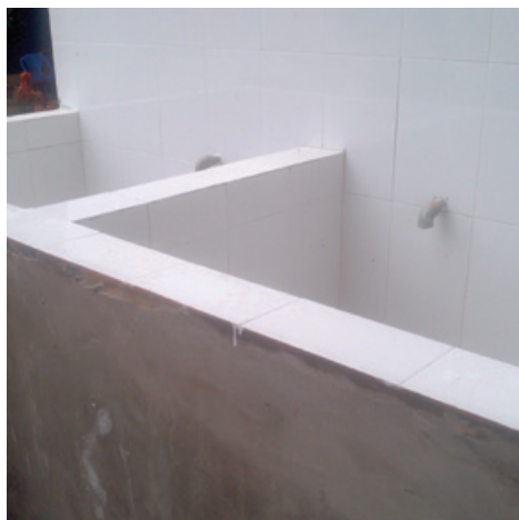
Dunk tanks for cleaning and disinfecting transport cages.
