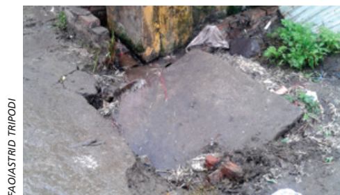
Drains that are easily blocked with organic material.
