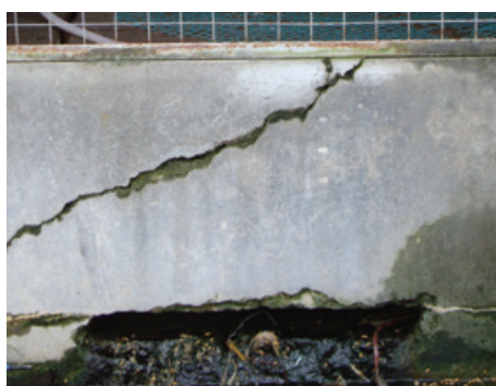
Drains and facilities in need of repair.
